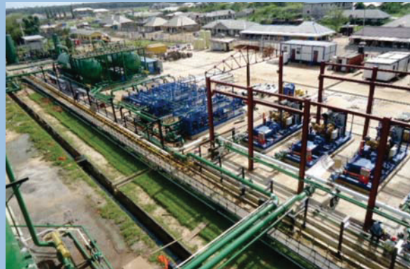
Aerial View of Liquid Treatment Facility
